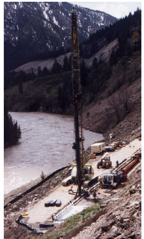
Micropile drilling operation.
