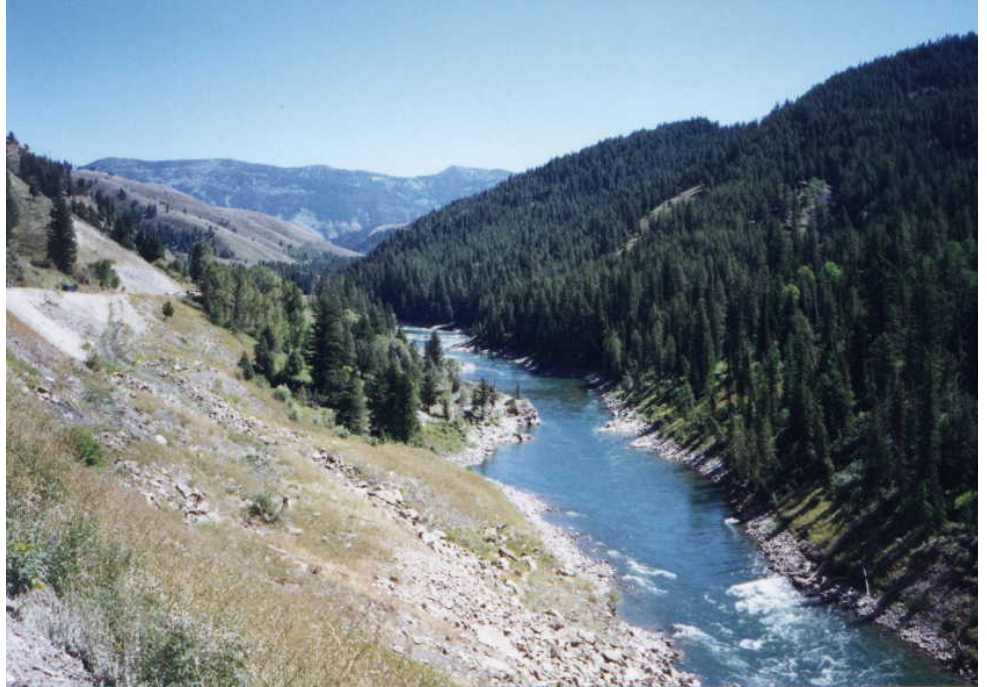
Pre-construction photograph showing the physical constraints at site.
