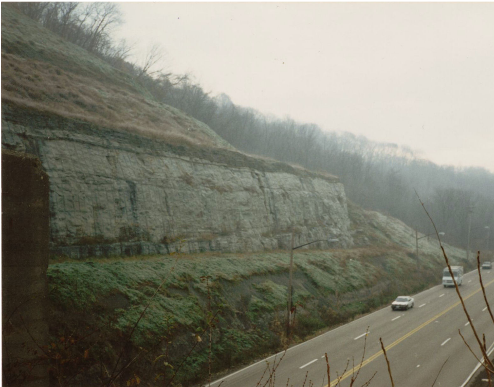
Rock slope following completion of D'Appolonia designed repairs.
