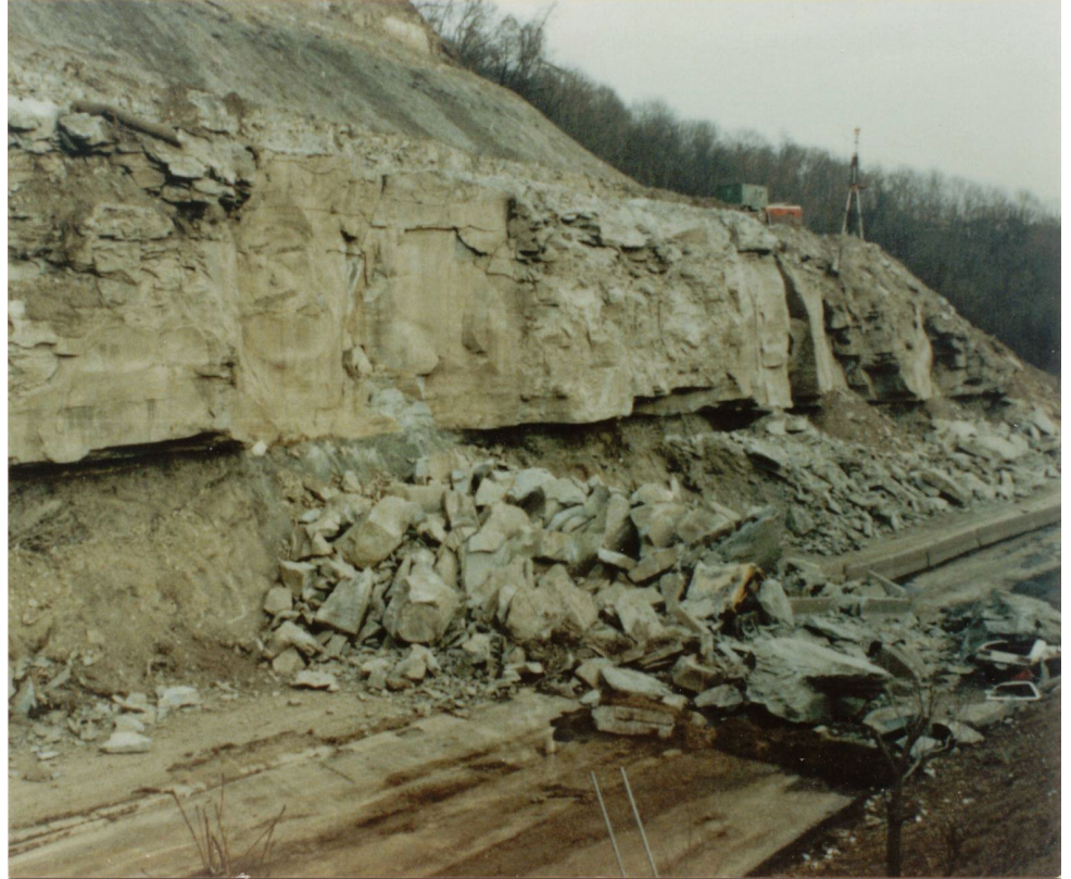
One hundred-foot-high rock slope along Saw Mill Run Boulevard following failure.
