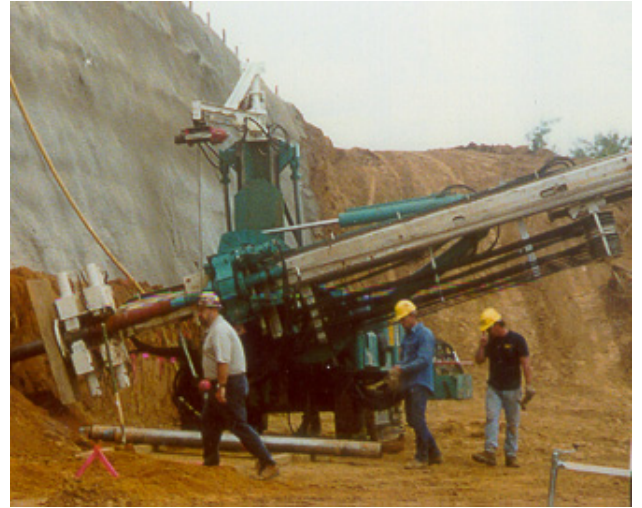
Soil nail installation at Natchez Bluff site.
