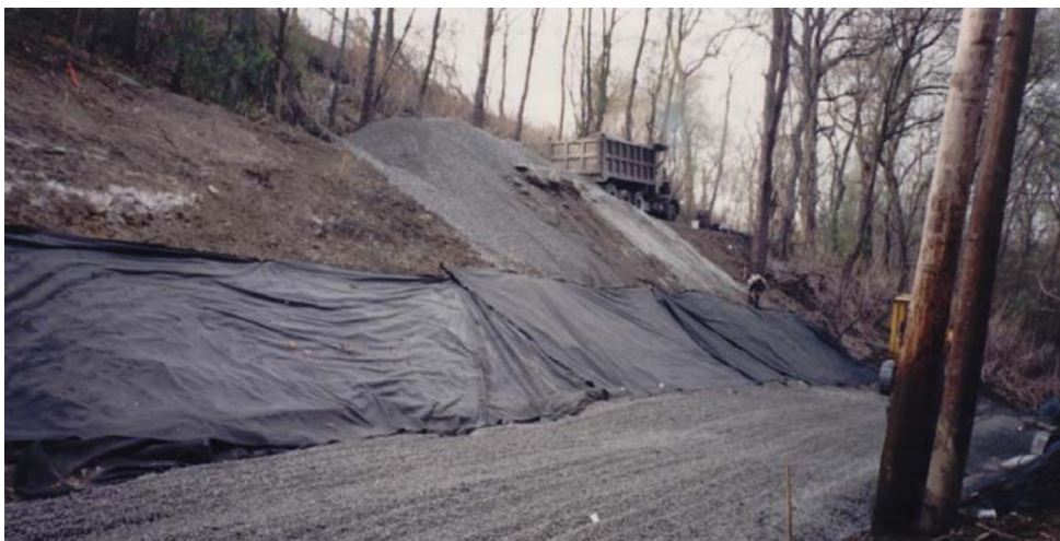
Reconstruction of 160-foot-long section of failed reservoir embankment.
