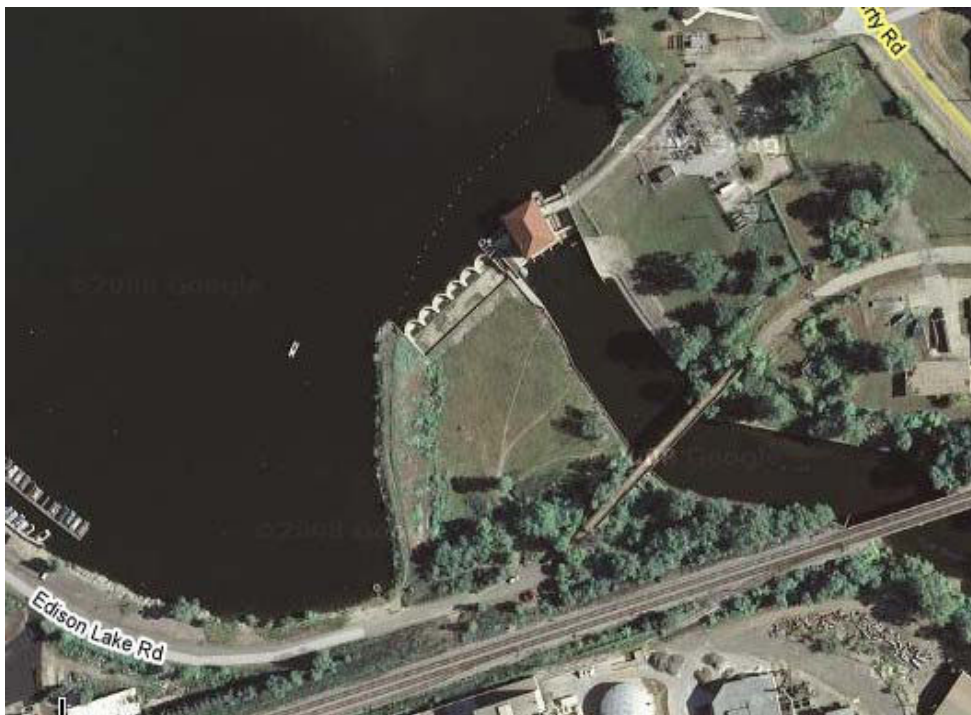
Aerial view of the French Landing Project on the Huron River in Michigan.
