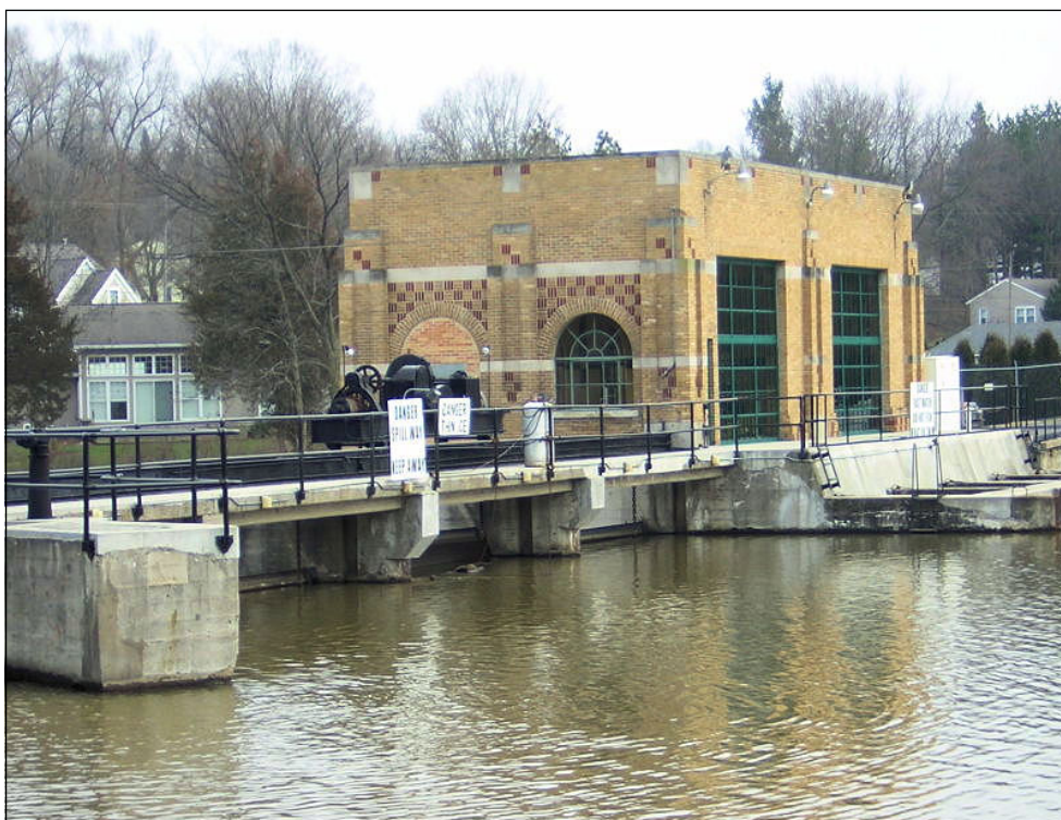
Powerhouse and spillway at Cascade Dam on the Thornapple River in Michigan.
