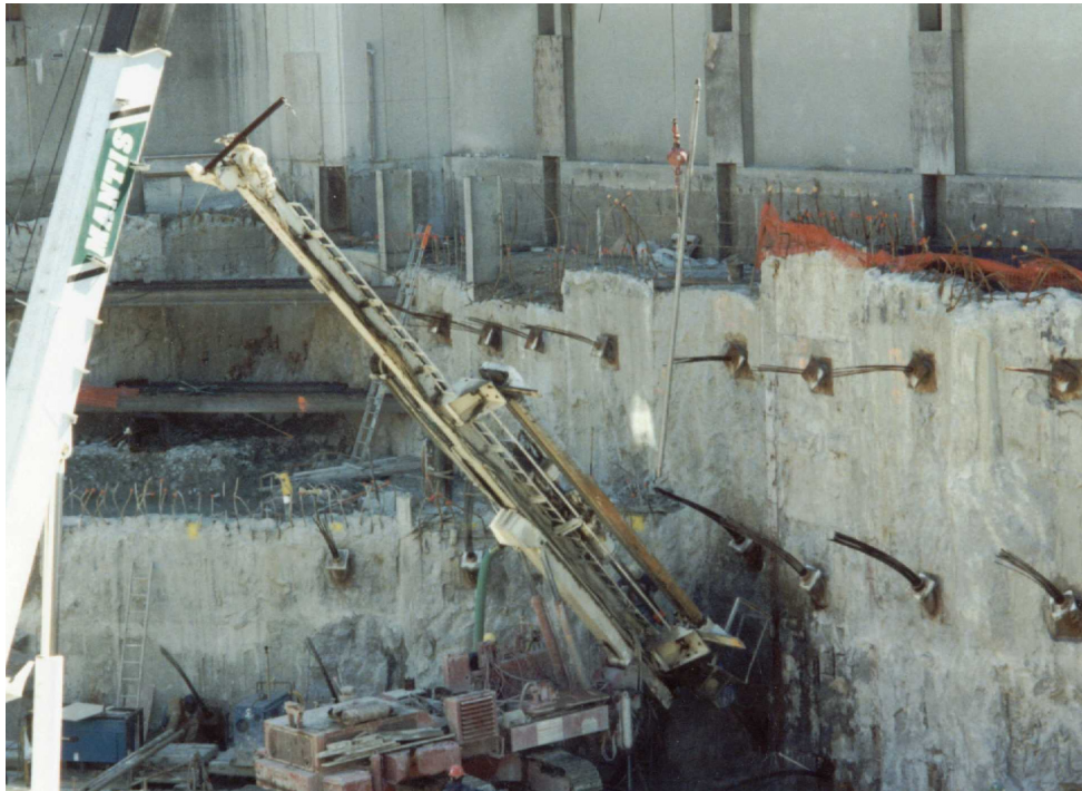
Drilling associated with inclined anchor installation at Cambridge Hospital.
