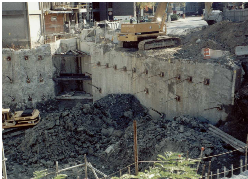
View of foundation excavation with anchored diaphragm wall in place.
