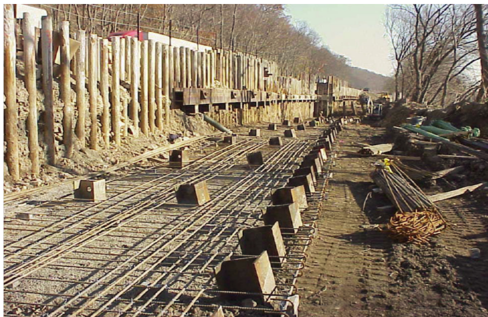
PADOT photo of retaining wall construction along the Juniata River.
