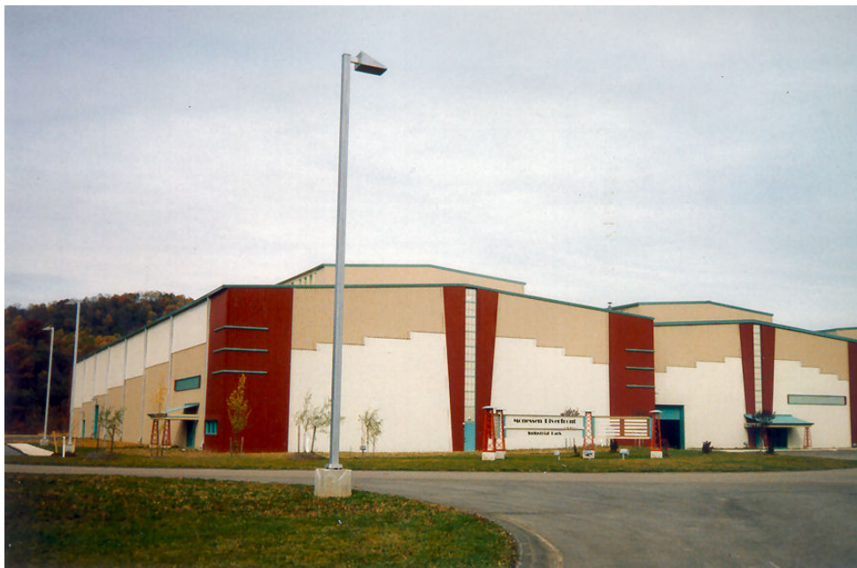
Monessen Riverfront Redevelopment Project after completion of initial phase.
