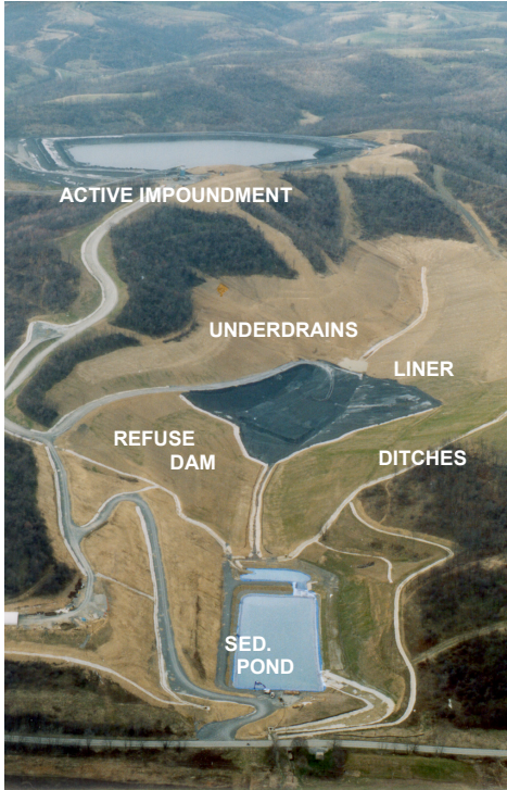
New site development (foreground) and active impoundment operations (background) are addressed.
